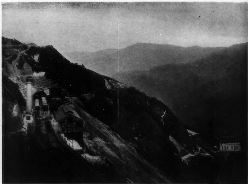
CABLE HOISTS, SÃO PAULO RAILWAY, SERRA DO MAR, BRAZIL
